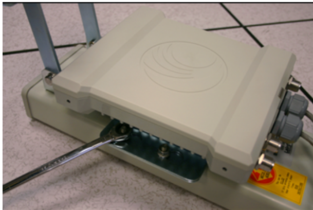
Figure 136: Lower bracket attached to AP antenna
