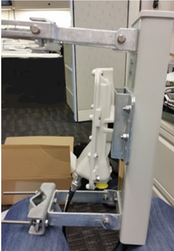
Figure 127: Completed AP and antenna assembly
