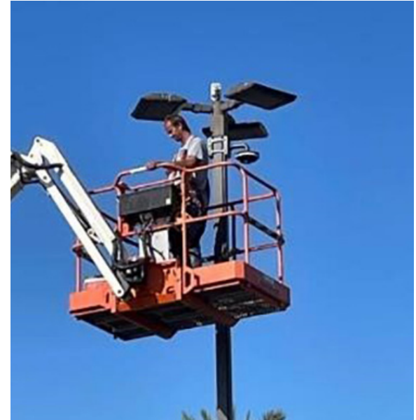
Field install of Bridge-in-a-Box for camera installation.
