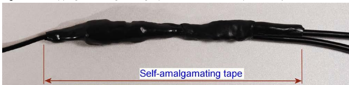
Figure 114 Wrapping self-amalgamating tape around the GPS adapter cable joint
