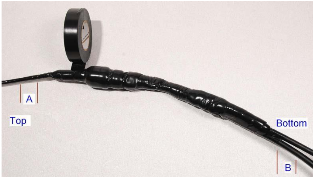
Figure 115 Wrapping PVC tape around the GPS adapter cable joint
