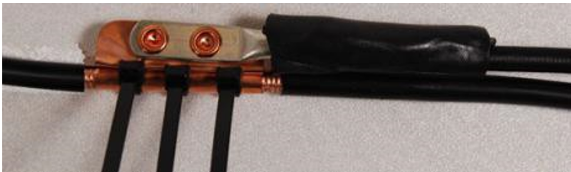
Figure 67 : Folding the ground wire strap
