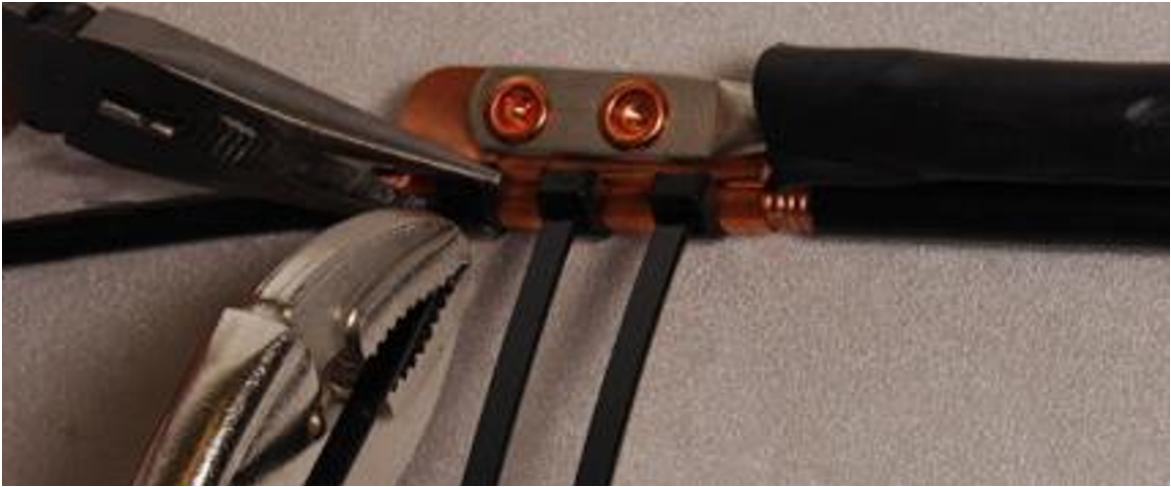
Figure 68: Tightening the cable
