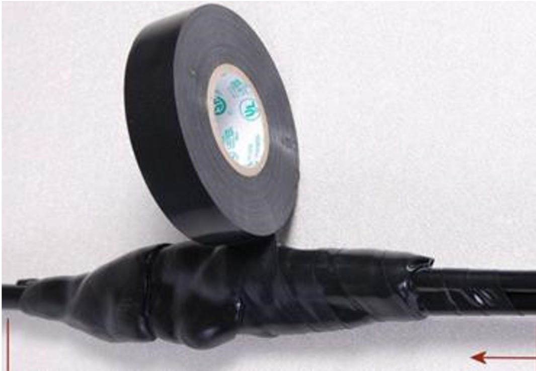
Figure 71: Wrapping a layer of PVC tape
