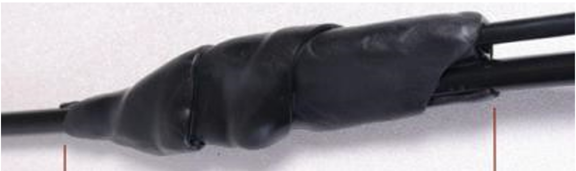
Figure 70: Wrapping the complete assembly
