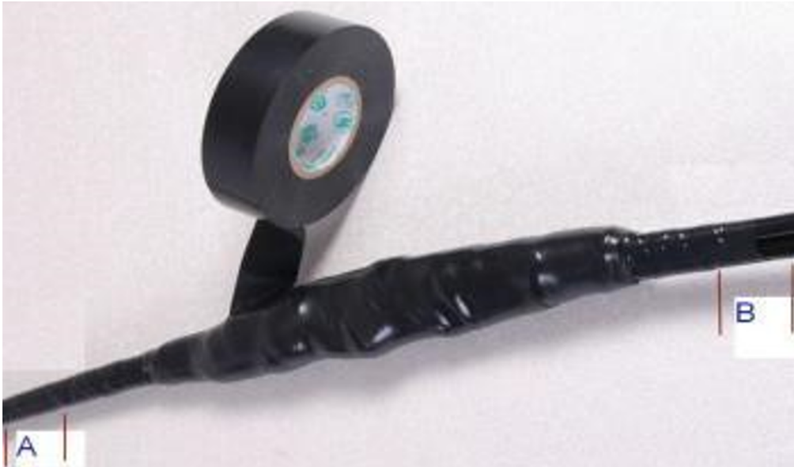
Figure 72: Wrapping the four layers of PVC tape
