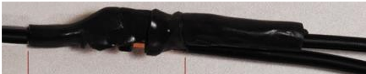
Figure 69: Cutting the self-amalgamating tape
