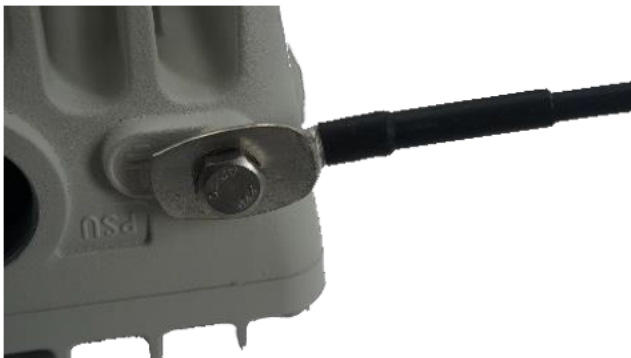
Figure 86: Fastening the copper ground cable
