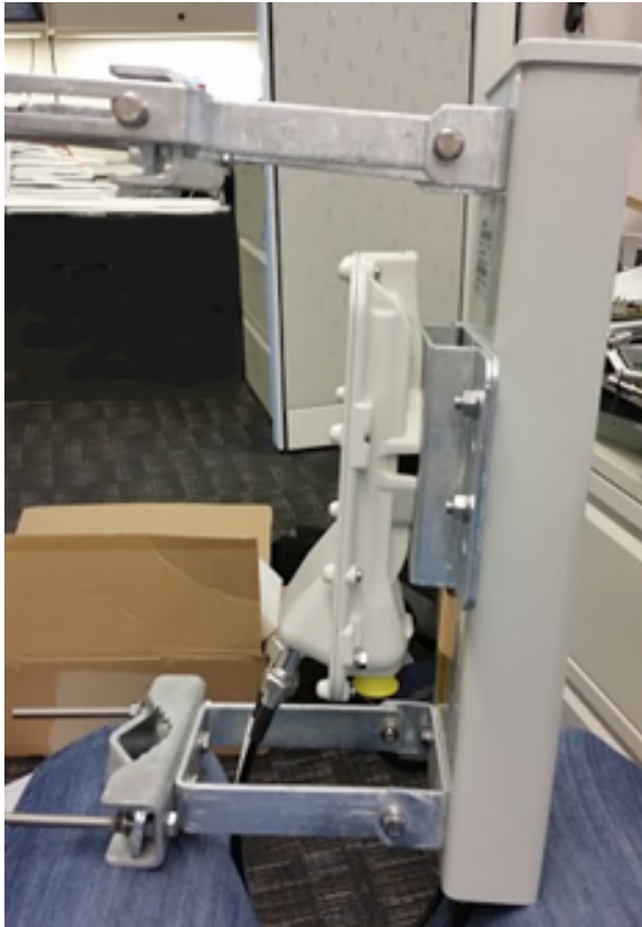
Figure 128: Completed AP and antenna assembly
