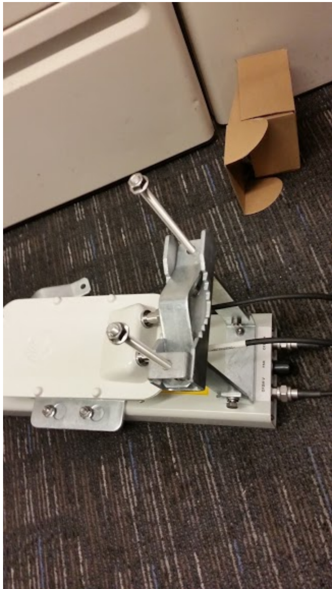
Figure 127: Lower bracket attached to AP antenna
